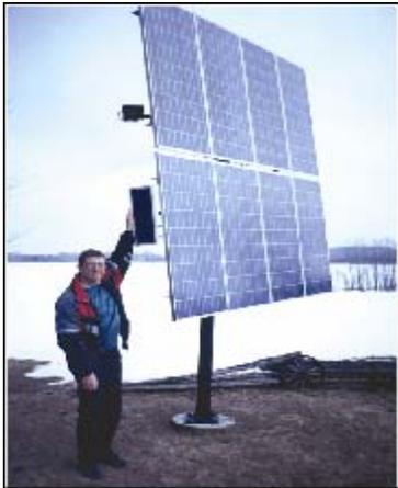
On bright cloudy days the PV array will take advantage of dispersed light by facing south. On dark rainy days the tracker will not move when there is no increased advantage in power output. This is a single axis tracker that uses unique circuitry and photovoltaic technology to sense the direction of maximum power output.
